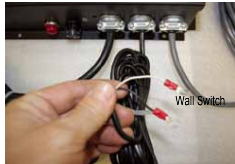
Figure 20a. (Remote Switch Wire connection)
