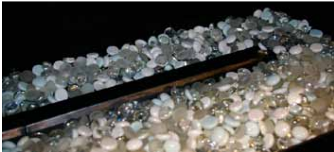
Figure 23. Completed glass bead installation. (Note: place glass beads on top of mesh pilot cover.)
